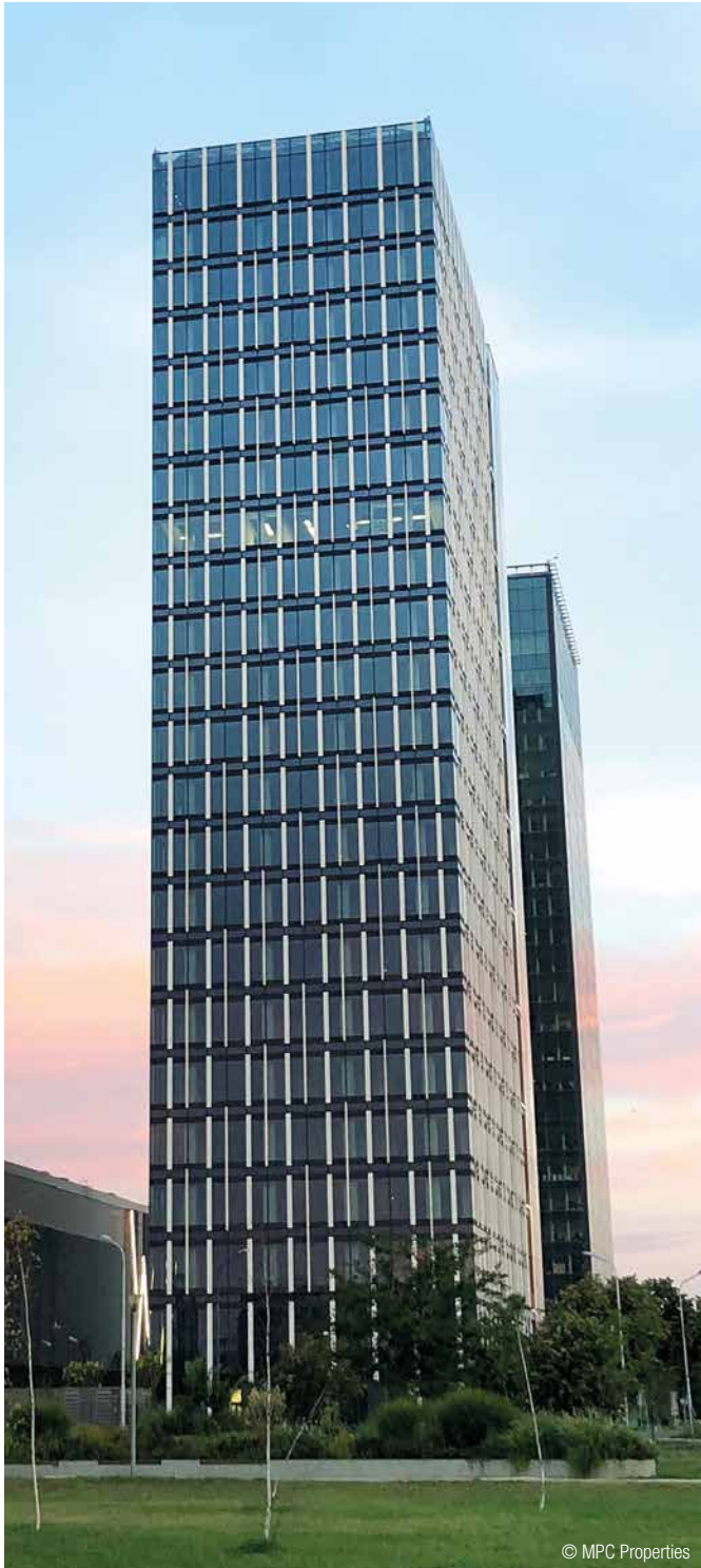
Ušće Tower two.
